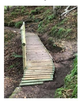
c. The damage to railings was not as significant as feared. A number of posts, railings and part of the top rail were replaced and reinforced.
