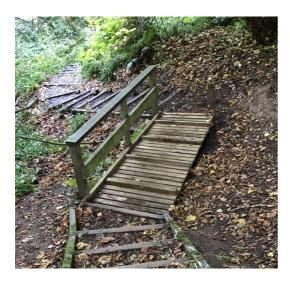
b. The damage to the second bridge was concentrated at the ends of the bridge and railings. Repairs were made to the decking and railings, and the decomposing leaves were removed from below the decking to encourage air flow and allow the piers to dry out more quickly. The removal of leaves will become an enduring maintenance task.
